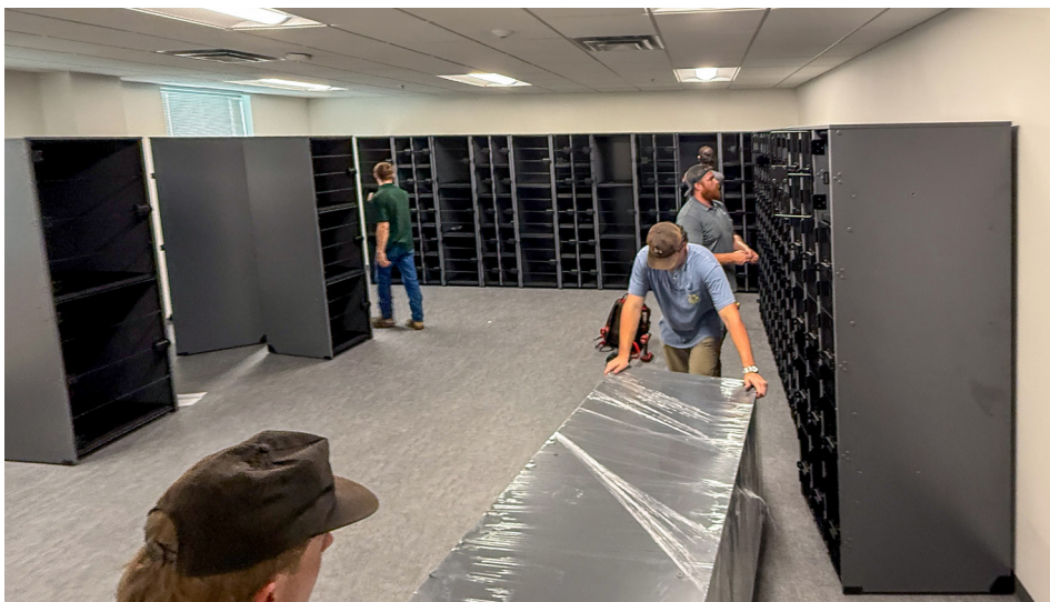
Fully assembled cabinets reduced installation time, labor, and cost.
